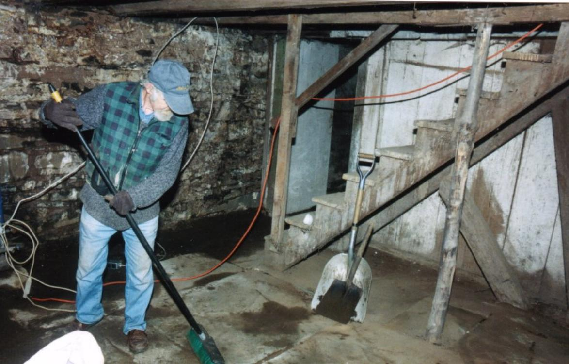
All debris was removed from the basement which revealed a bluestone floor.
