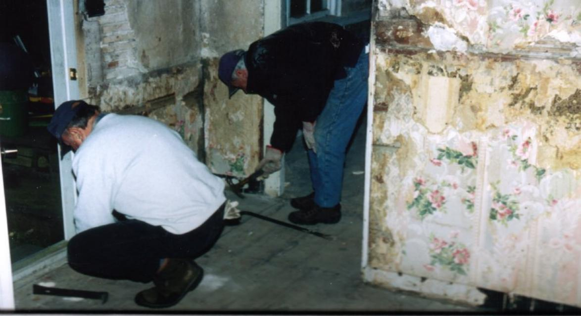
Several layers of floor coverings were removed to expose original wood floors.
